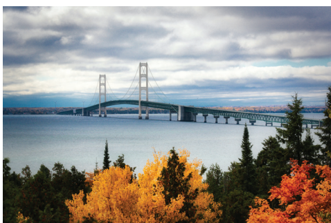
The Line 5 pipeline runs directly through the Straits of Mackinac, transporting up to 540,000 barrels of oil per day.
