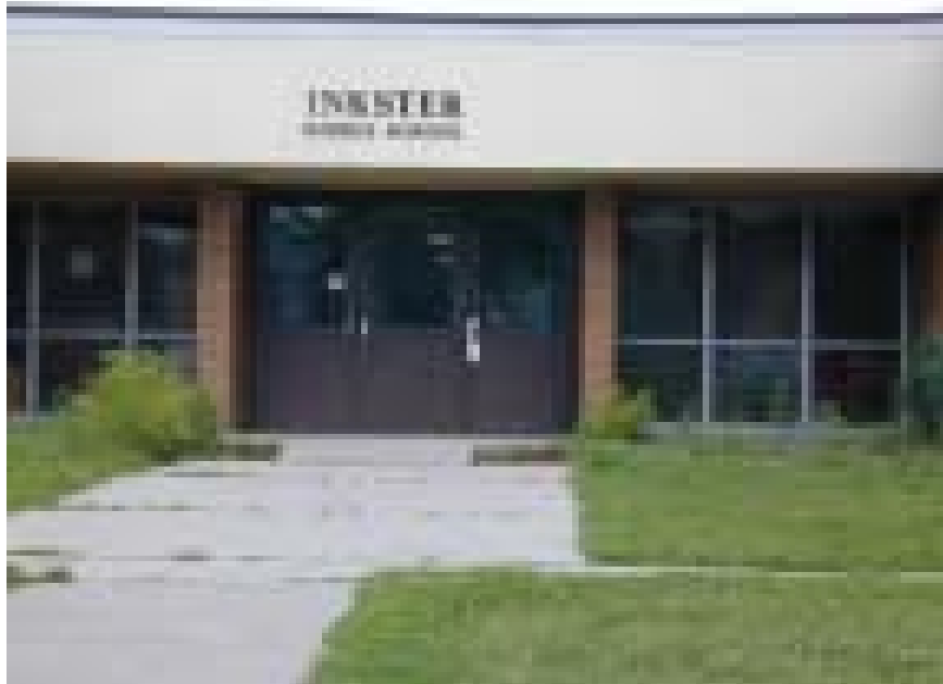
This dilapidated building houses the Inkster Middle School. It is one of several failing schools in the district that will be taken over by Edison Schools Inc., a private company with a track record for building successful schools.
